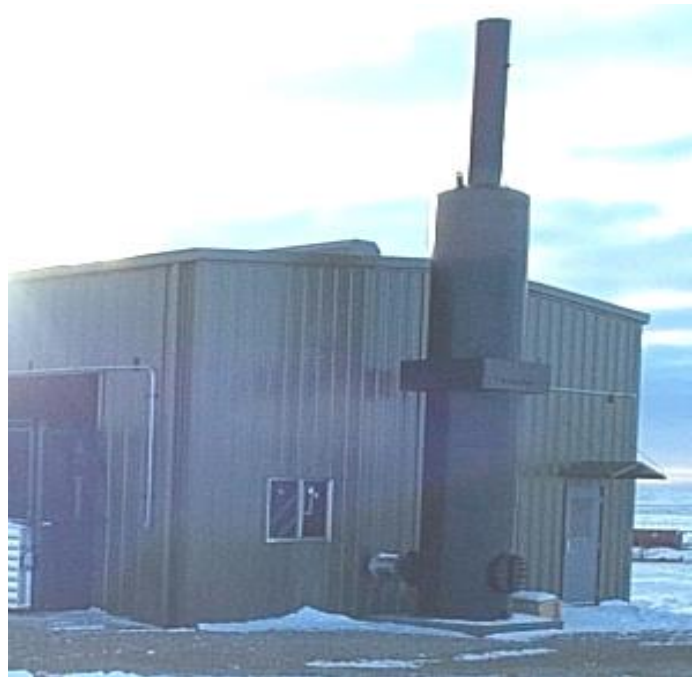
Figure 10: Oxidizing Converter with a DPC-2804LE
